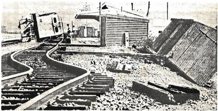
THE EARTH ALSO moved underneath Edgecumbe's railway station, with leaning buildings, a toppled engine and a crooked railway line giving some indication of the full force of the quakes.
