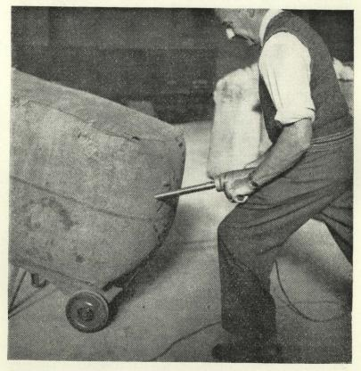
Fig. 3-Drawing a core sample from a bale of scoured wool.
