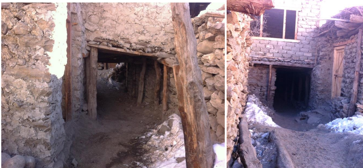
Plates 10 Tunnels in Hushe
