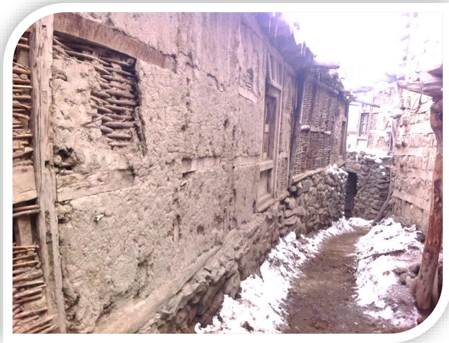
Plates 8 Traditional wall of a house in Prono, made up of mud and clay.
