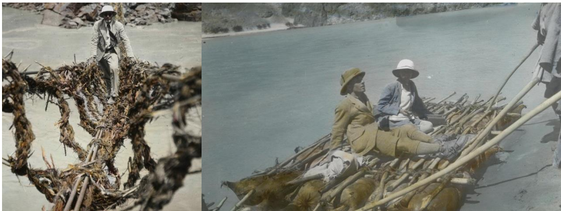
Plates 4 Kharmang bridge Crossing (Left) and Ferry Crossing in Baltistan (Right) in 1940. Photo by Ralph R Stewart
