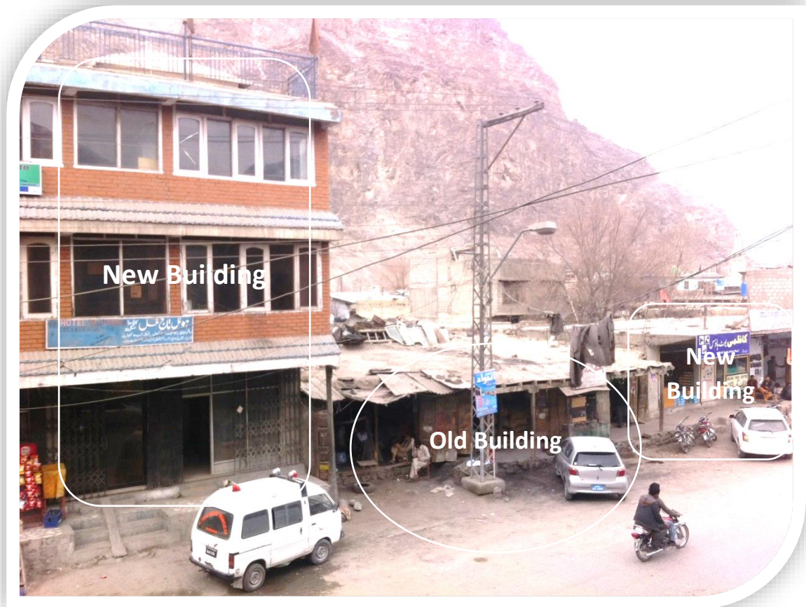
Plates 20 The picture shows a modern three-story building next to some old traditional shops (Skardu)
