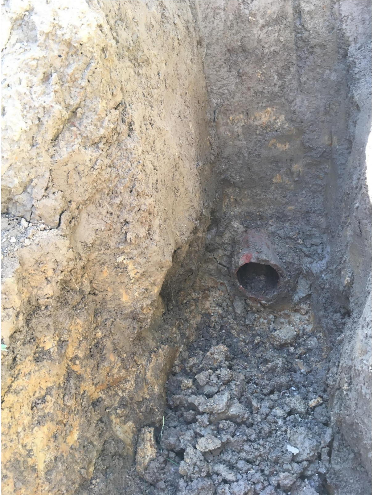
Plate 4-6. The excavated, ca 13.5 cm diameter, tile drain at the catchment outlet could be identified from hyperbola reflections on the GPR radargram. The clay pipe was found at a depth of 70 – 80 cm and can be seen to be overlain by a well-structured fill, including topsoil.
