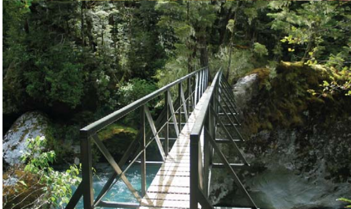
Figure 4.1g-7: is a bridge installed recently across the lower Beans Burn. Prefabricated and brought in by helicopter the installation team have subsequently struggled to make it fit the physical site.
