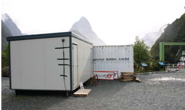
Figure 4.1c-9: Construction-related facilities. Note the tape holding the electrical wire in place on the near face of the structure.
