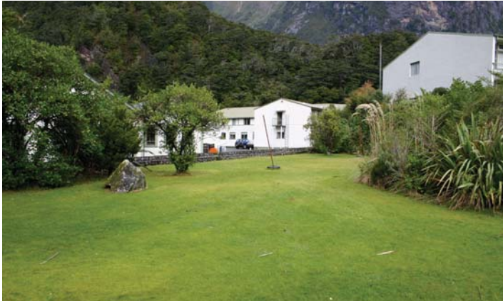
Figure 4.1c-1: Dilapidated post-war buildings and closely mown lawns around the hotel. Indigenous forest is in the background.
