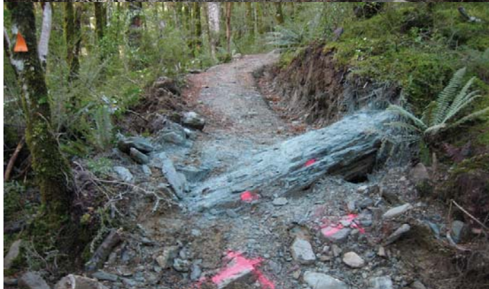
Figure 4.1g-11: show the pink paint marks where drill holes have been made so rocks the digger was unable to dislodge or break up can be shattered by explosives.
