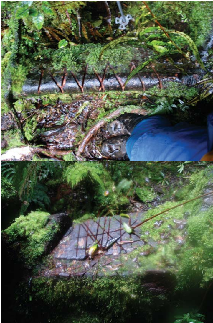
Figure 3.6b: Steps made in roots of a tree, with crosshatched grip cut by chainsaw. Such 'facilities' are not included in the VAMS inventory
