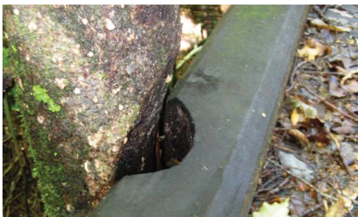
Figure 4.1c-20: Detail of the visitor walkway to the passenger terminal. In this image both the timber and tree have been rebated to accommodate each other. Note the timber used in the walkway is an imported Pacific hardwood.
