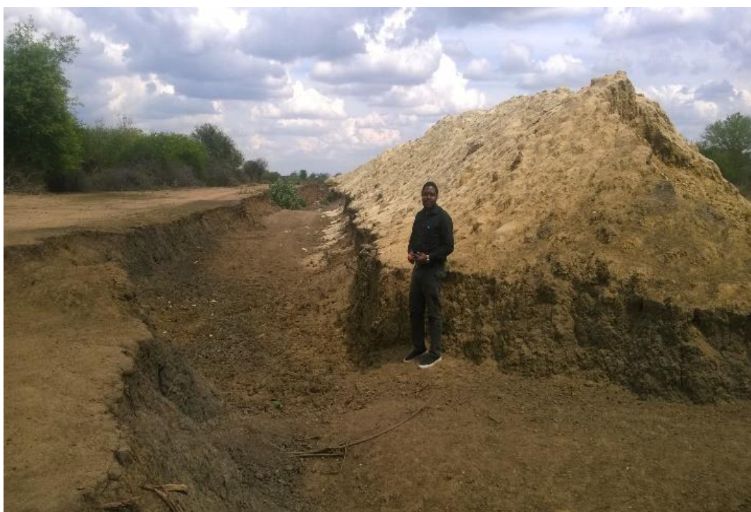
Plate 5.1 Excavated trench and heaped soil between Kambala and Dihombo Villages
