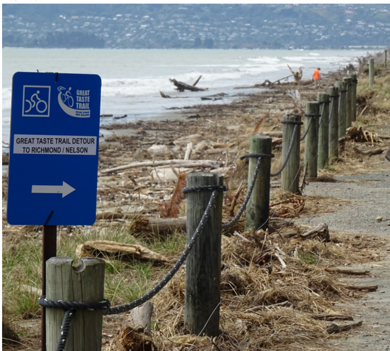
Damage from Cyclone Gita, Moturoa/Rabbit Island, Tasman District.
