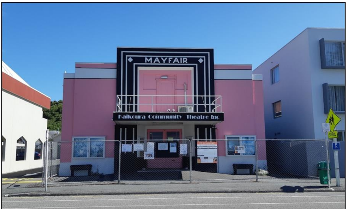
Figure 15: The damaged Mayfair Theatre (Author's image)
