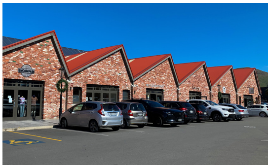
Figure 39 Saw-tooth roof of The Tannery (image by author).
