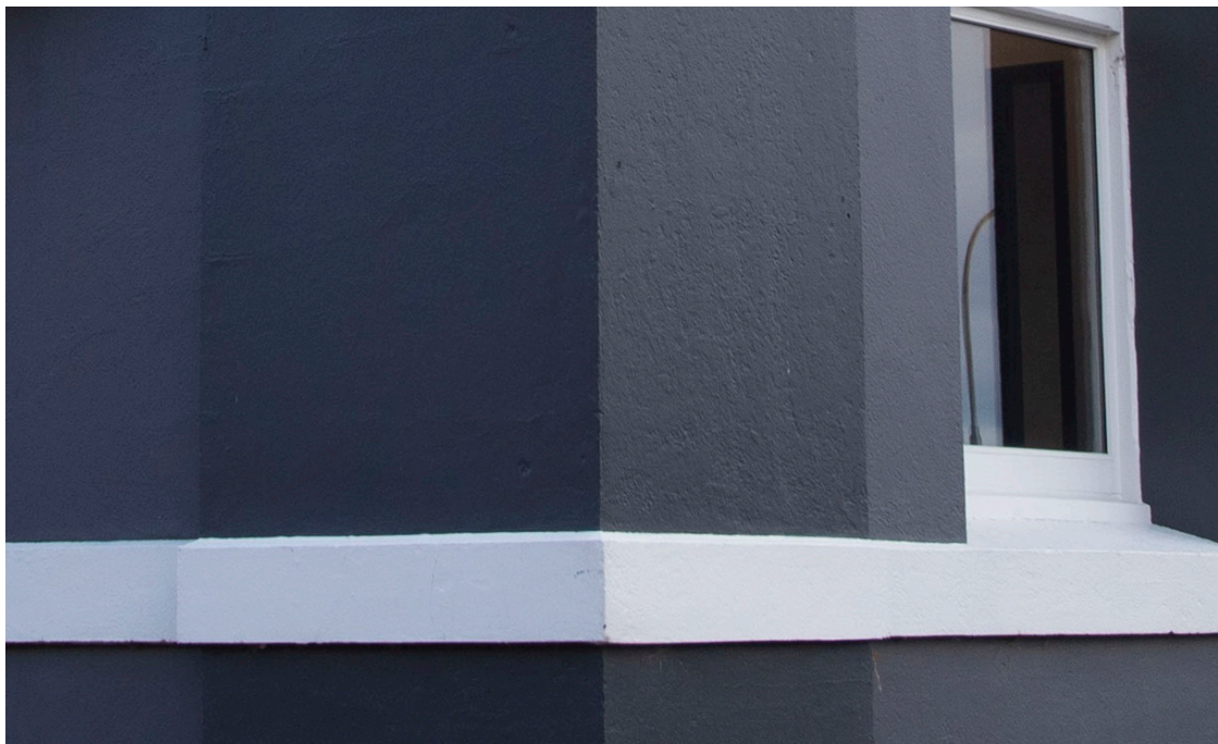
Figure 77 Relatively smooth concrete surface in Dunedin Warehouse Precinct (image by author).
