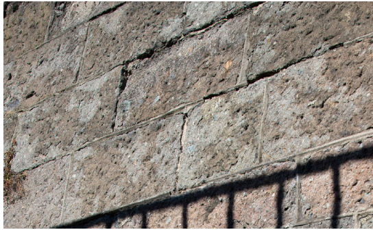
Figure 75 Rough stone surface on railway overbridge in Dunedin Warehouse Precinct (image by author).
