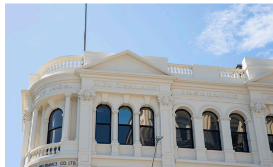
Figure 38 Decorative cornices and double-hung windows found on former New Zealand Insurance Company building (image by author).
