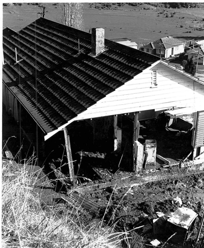
Fig. 7 Damage caused by a debris avalanche in Kiwi soils.
