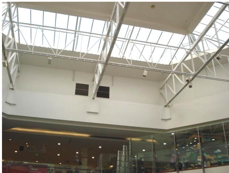
Figure 47. St Lukes Shopping Mall in Auckland uses skylights to let some natural light into the mall (Source: Author)
