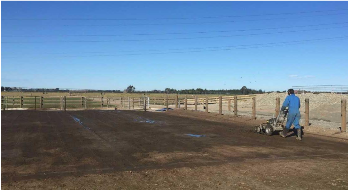
Photograph 1: Geotextile carpet being cleaned using motorised rotating brush sweeper.
