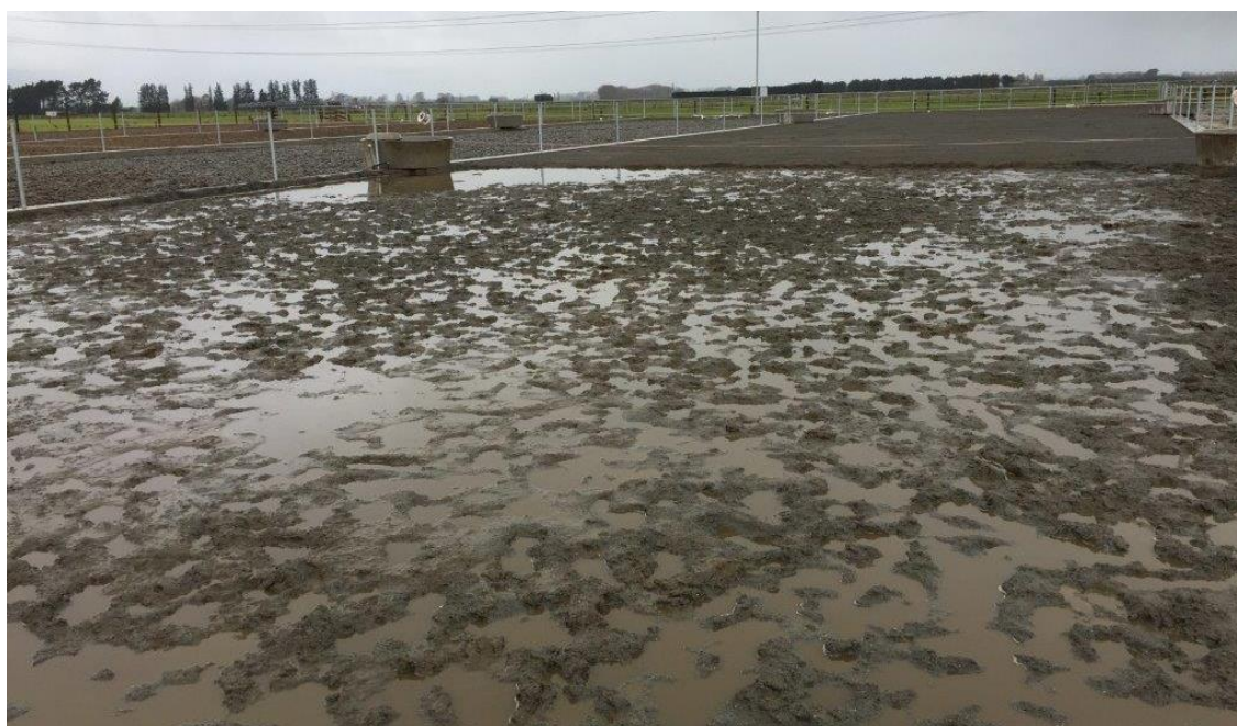
Photograph 5: Sand stand-off area with extensive surface ponding after heavy rainfall in July. Area is fenced to achieve 10m 2 /cow stocking rate and area behind the tape is unstocked.
