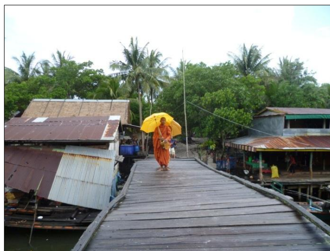
Figure 5.3 A young Monk crosses over the Prek Svay River Bridge
