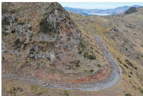
Figure 1 Rockfall impacts Summit Road on the main Port Hills ridgeline following the 4 September 2010 and 22 February 2011 earthquake events (photo kindly provided by Graham Hancox, GNS Science).
