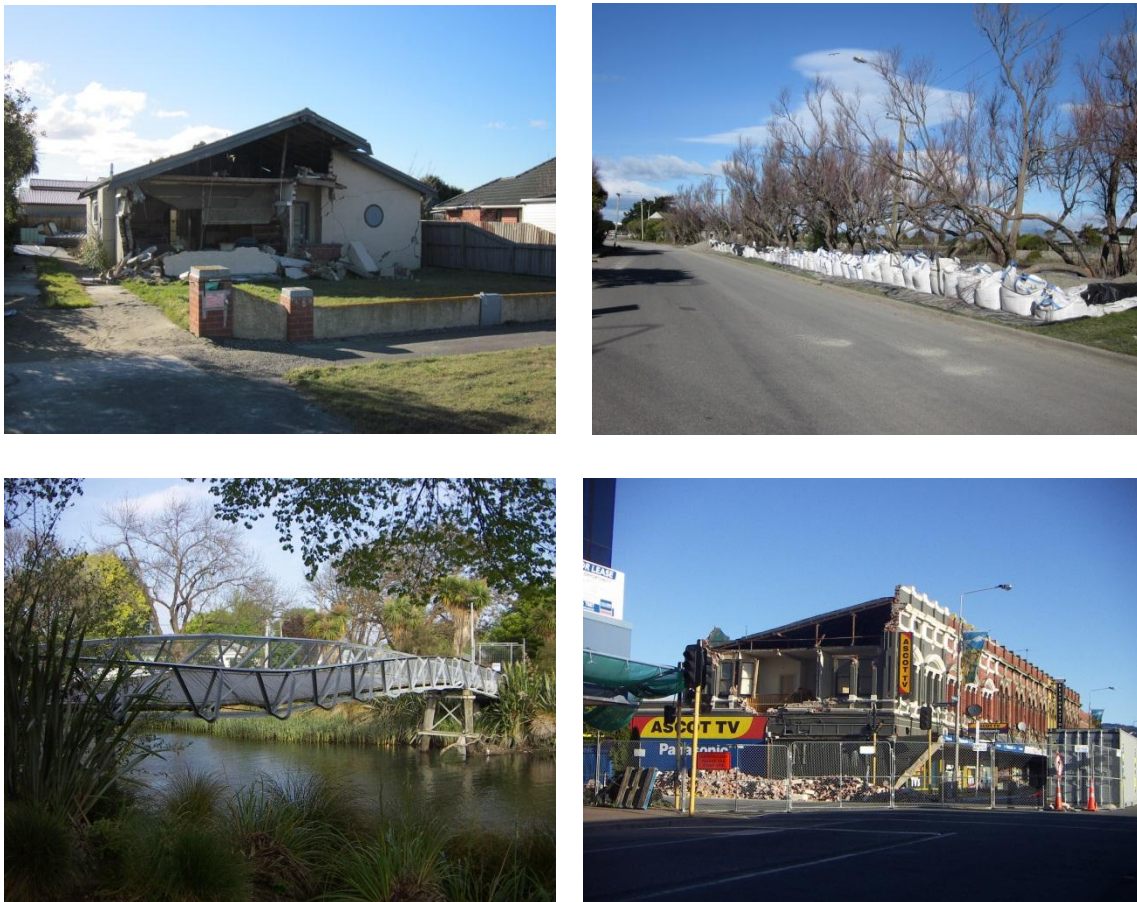
Figure 1: Damage to housing, river banks, infrastructure and suburban centres
