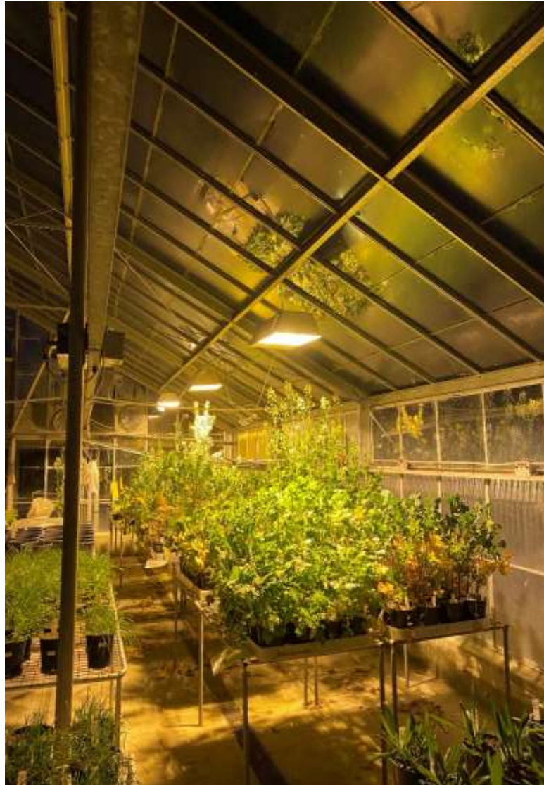
Figure 3.1 Supplementary light provided by sodium lamps for artificial 20 hour photoperiod in glasshouse at Lincoln University, New Zealand.
