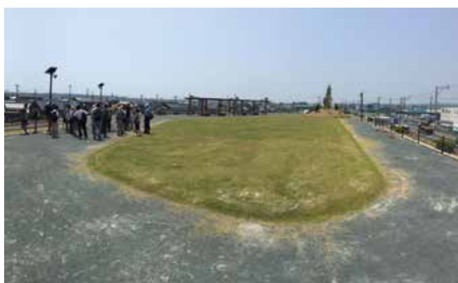
Figure 1. Heisi no inochi-yama , a tsunami evacuation mound built in 2012. (Photo credit: Carol Smith)
