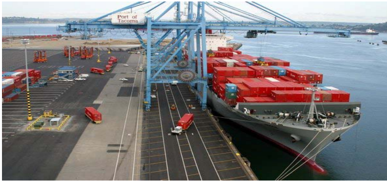
Figure 2.3: Quay Crane at the Port of Tacoma, USA
