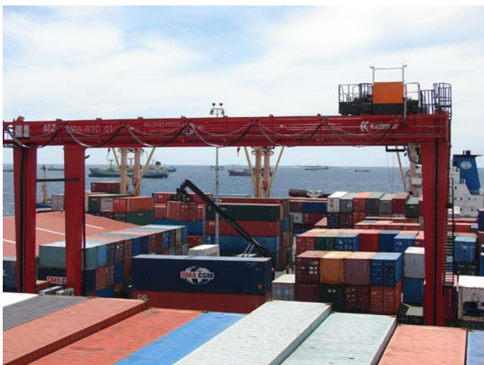
Figure 2.4: Yard Crane at Male' Port, Maldives
