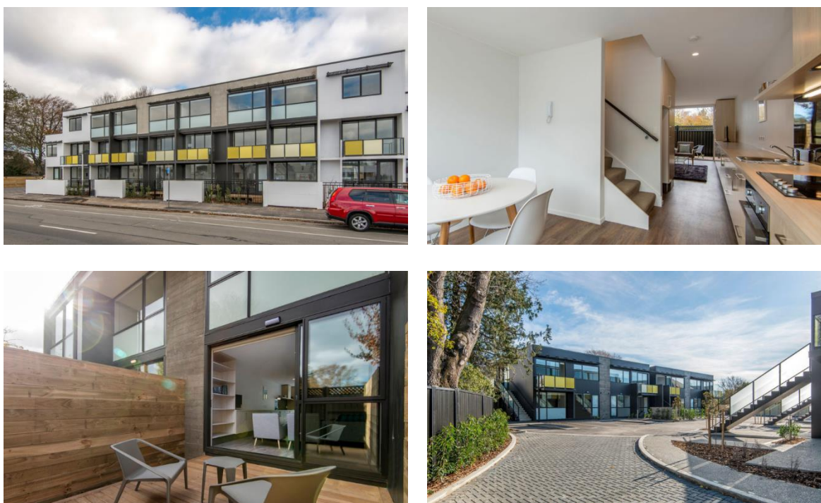
Figure 7 - 399 Manchester Street - Completed Development (Open2View, 2016).
