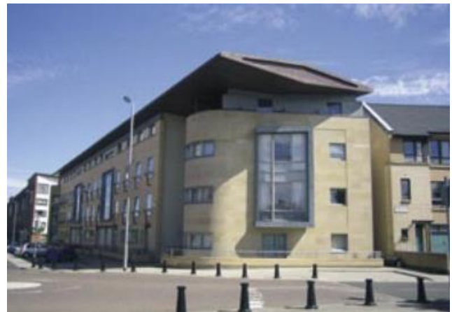
Continuous frontages with few blank walls
