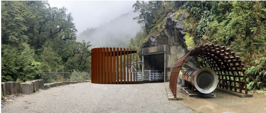
Figure 4: Preliminary design for the Memorial Pavilion at Pike River Mine. The proposed Pavilion, to the left, 'captures' the space emerging from the large, square portal – the entry to the long horizontal shaft of the mine. The Pavilion echoes the curved structure to the right, which protects the ventilation fan, and is made up of mine 'sets' usually used to hold up the inside of a mine shaft but here are deployed in the open air.
