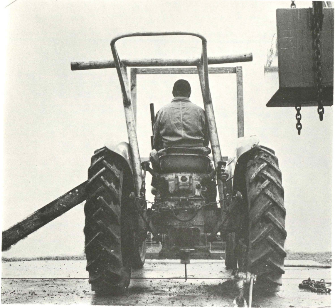
SAFE "T" SAFETY FRAME AFTER IMPACT FROM SIDE.
