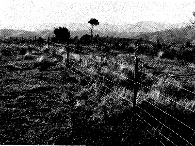
Curves and slight bends can be taken with ordinary standards.
