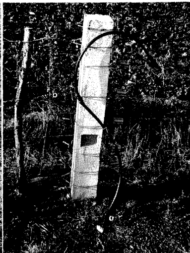
A wire threaded through a plastic pipe takes the live wire under a gateway. The earth wire must be taken across the gateway too. Plastic covered wire is often used satisfactorily under gateways.
