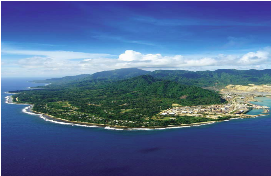
Figure 1.3: Aerial view of Niolam Island, the biggest island amongst the Lihir group. The gold mine operation is visible to the right. (Source:Bainton, 2006)
