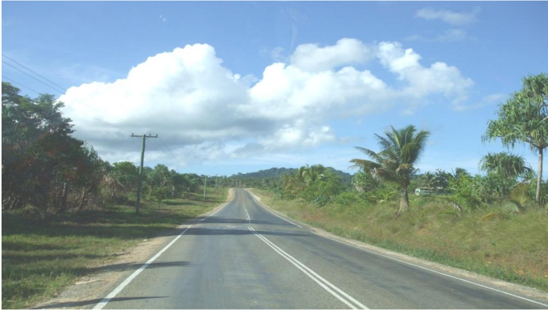
Figure 6.5: Part of an improved road system on Lihir
