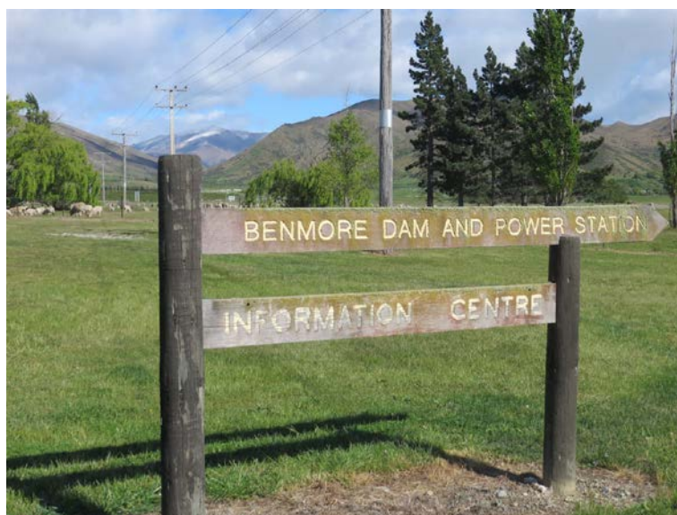
Photograph 31: Information centre sign showing wear and tear
