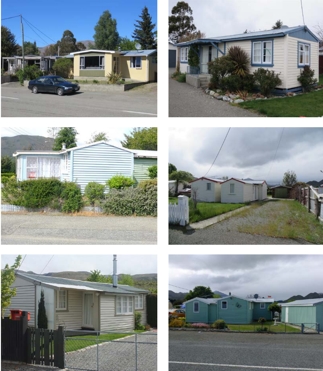
Photograph 7: Montage of Otematata T-Shape houses
